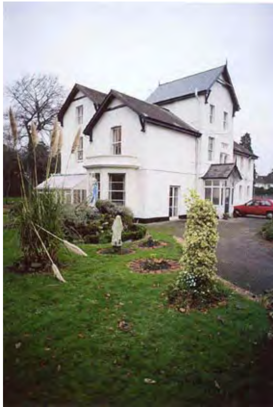
Wallace's house at Grays. The Thurrock Local History Society has (on the suggestion of the A.R. Wallace Memorial Fund) recently had it given Grade II listing on architectural merit.
