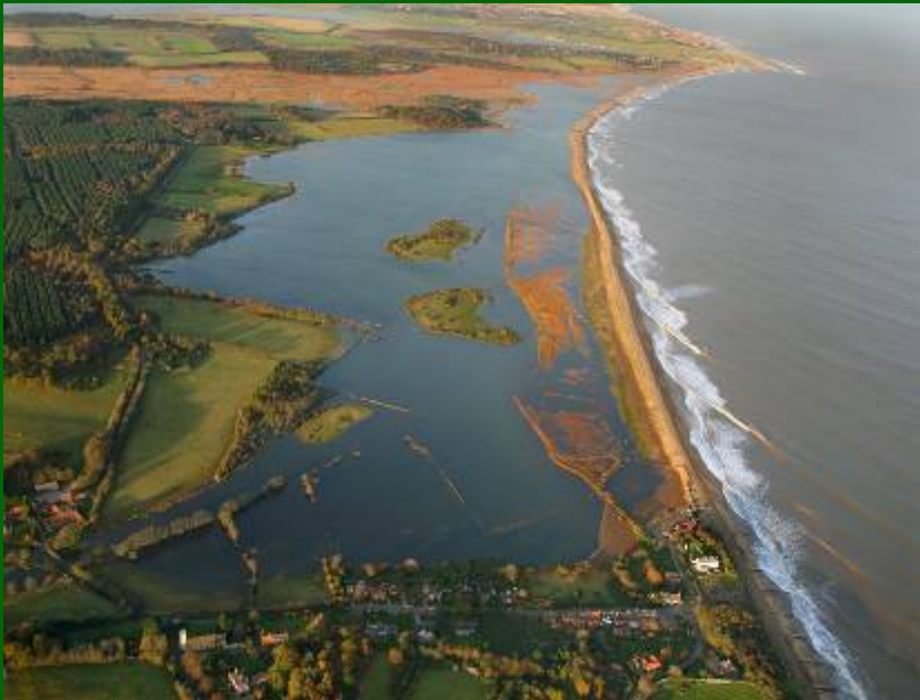
Sea wall breach - Dingle Marshes, Dunwich, Suffolk – Oct 07
